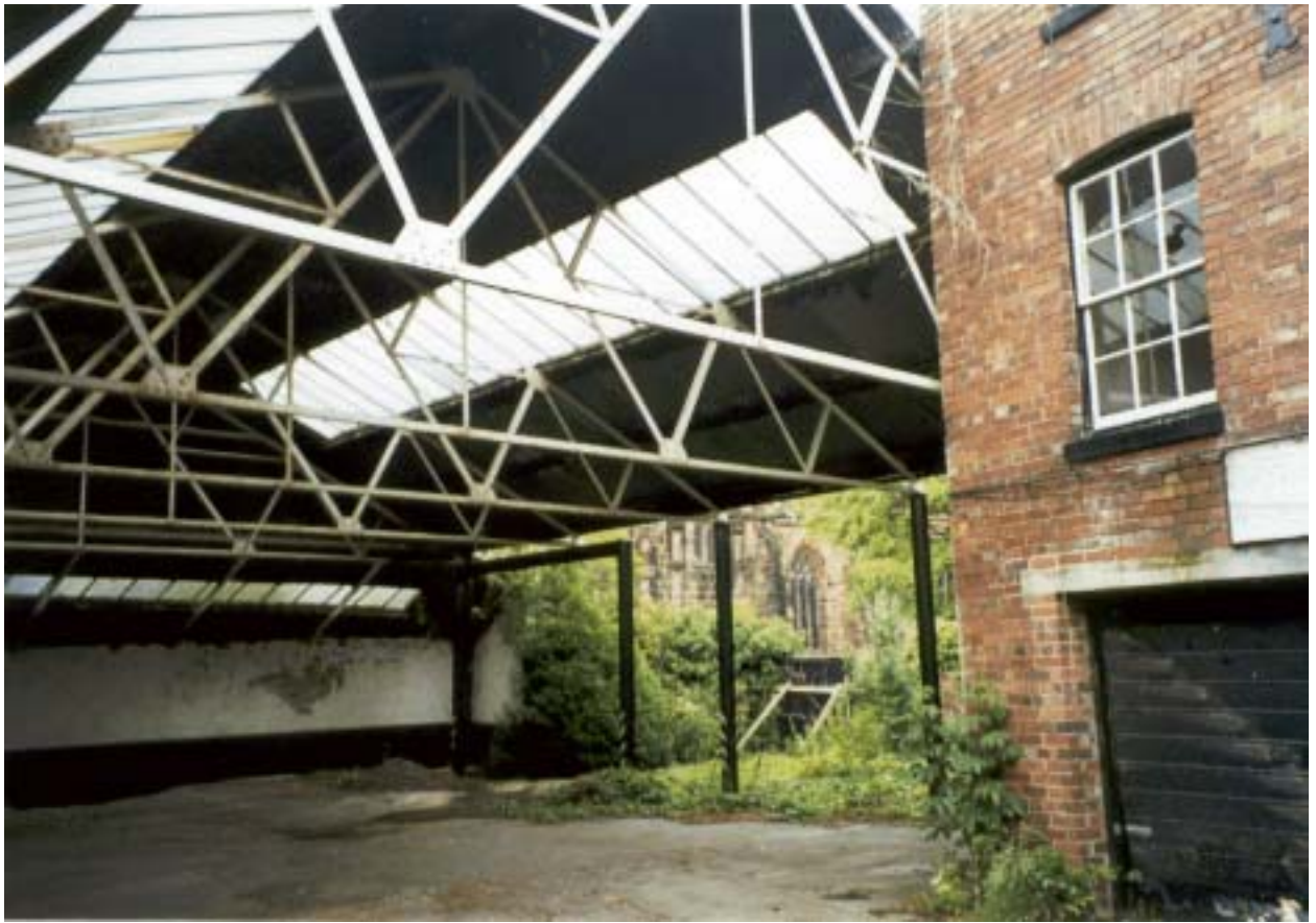
Metal frame shed in the courtyard
