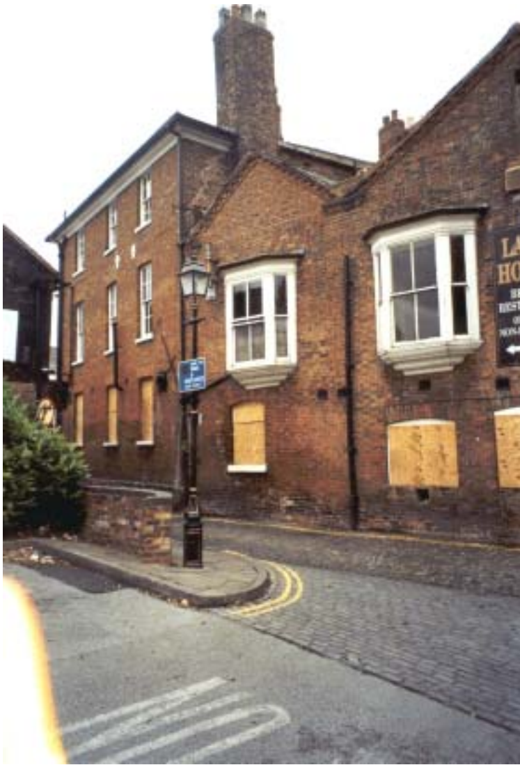
Church Lane: View from car park
