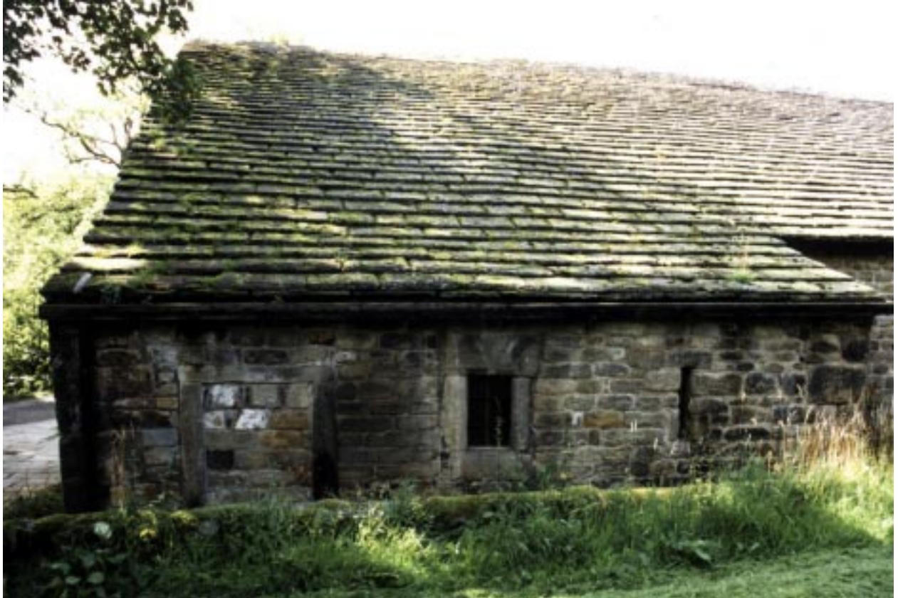
6. Blocked door in outshot probably gave access to feeding passage for cattle
